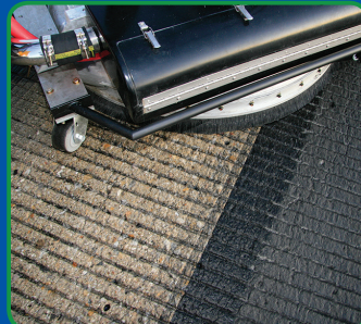
Cleans into the grooves of a runway for increased friction and drainage.
