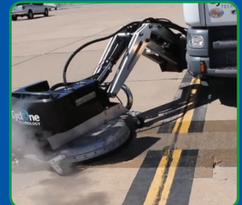
Single pass paint removal leaves surfaces clean and dry within minutes.
